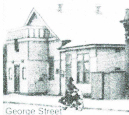
The Moe Mechanic's Institute Hall
