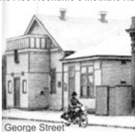
The Moe Mechanic's Institute Hall
